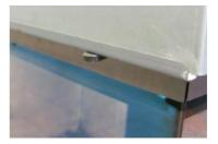
The front glass is released by wrenching the bracket below and above the side glass.
